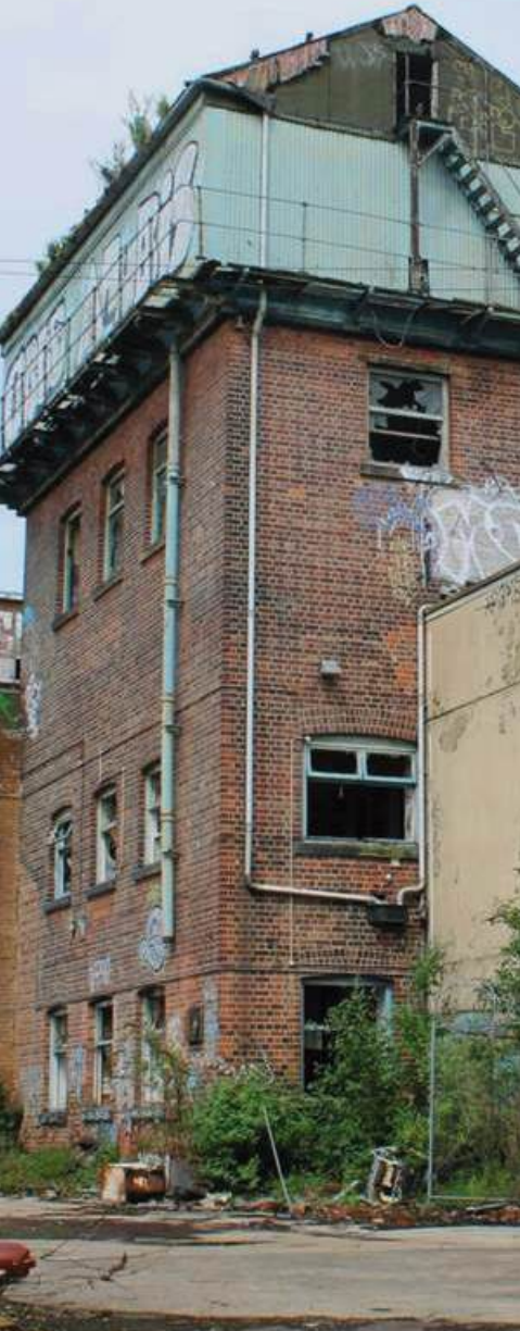
Water Tower, Stones Cannon Brewery
